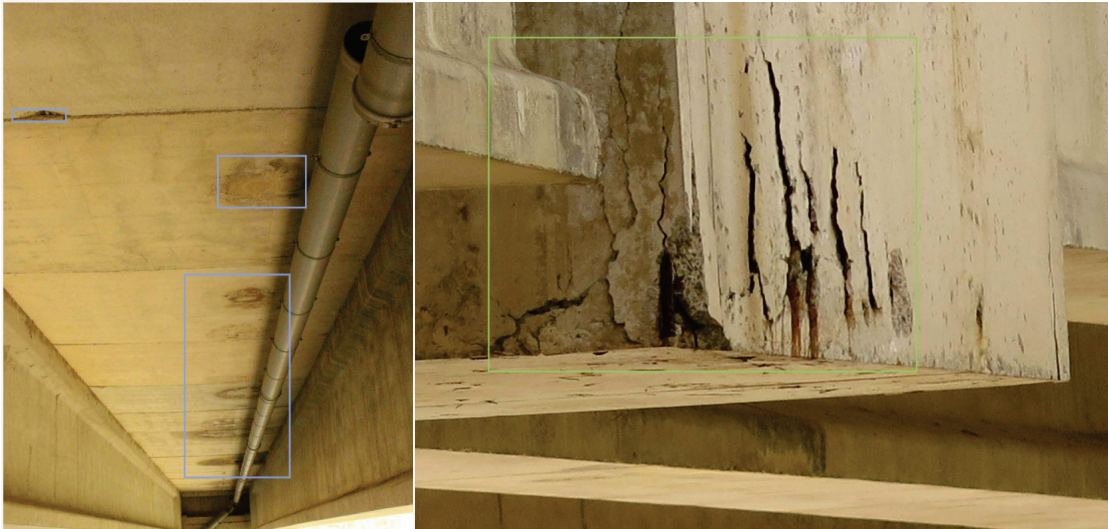
Figure 6a: Defects detected by the system's AI algorithm are marked out on the uploaded images
